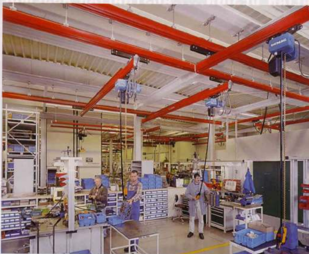
Staff can lift at the same pace all day every day with small workstation cranes. (Photo courtesy of Demag)
